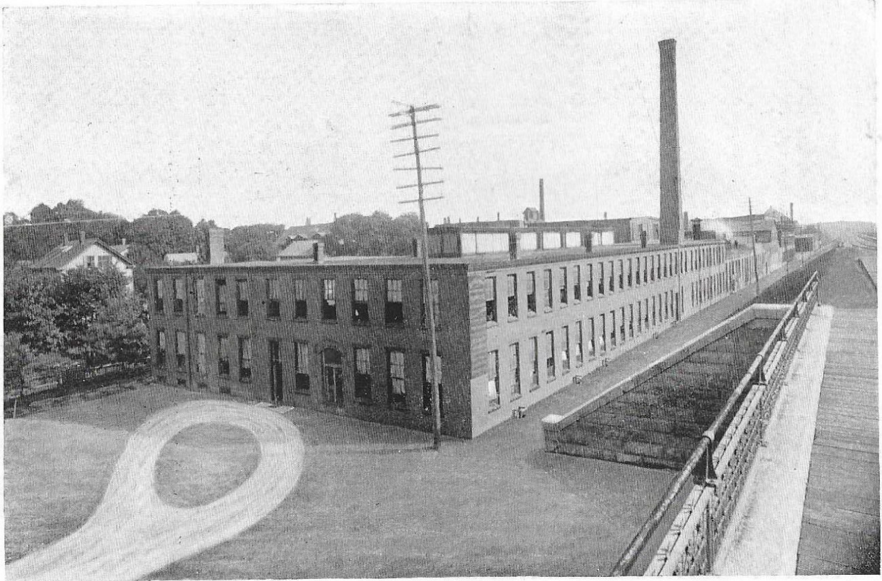
FIG. 49. VIEW OF B. F. STURTEVANT CO.'S WORKS, JAMAICA PLAIN, MASS., SHOWING RELATIVE SIZES OF CHIMNEY AND INDUCED-DRAFT PLANT STACK.
